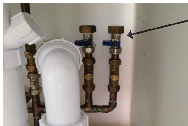
Washing machine valve under kitchen sink unit where applicable.
