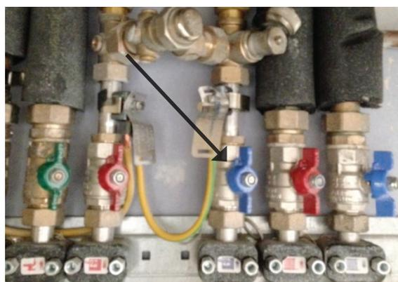
Radiator pipework valves above Heat Interface Unit
