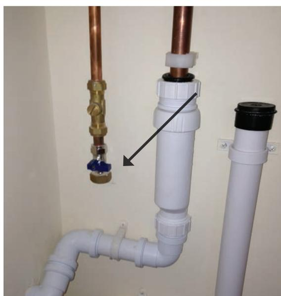
The washing machine valve is located in the HIU cupboard. Where a washing machine is located in the kitchen then the valve will be underneath adjacent to the appliance.
